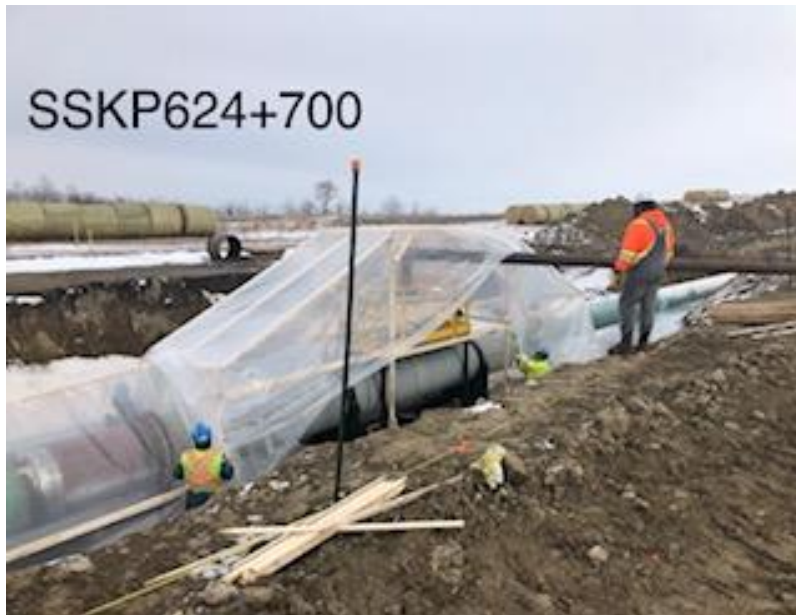
Banister crew members hoarding the test section
