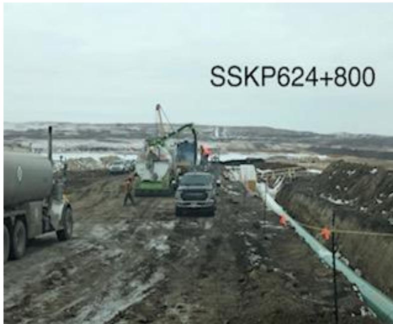
Setting up equipment at Chapleau Lake east
