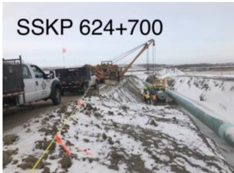
Test head in the main line ditch SSKP624+700
