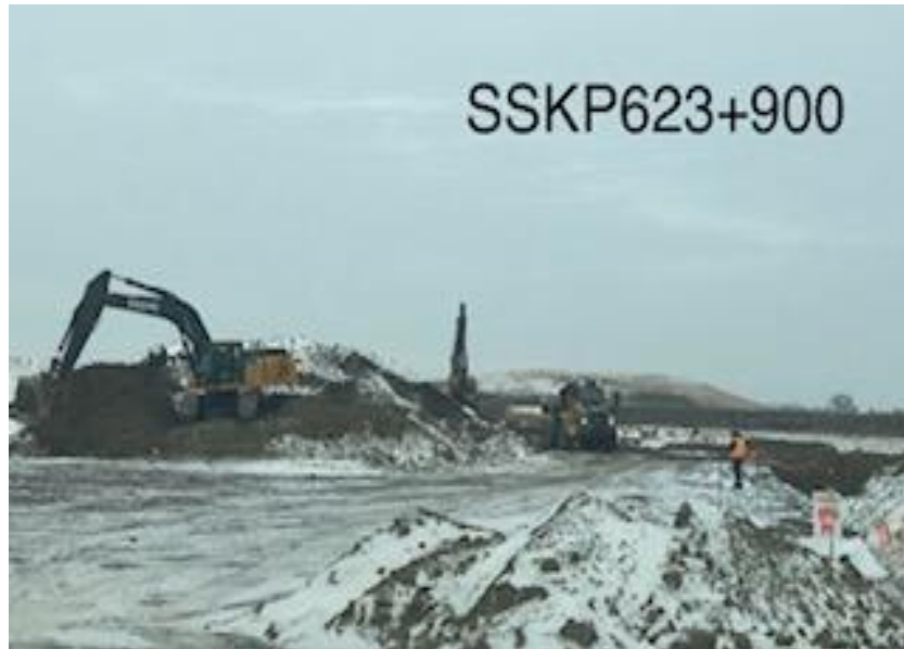
Backfill on west side of Chapleau Lake SK WC68
